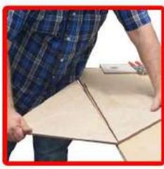
Diagonal cuts need a firm score, squeezing is possible if you are very gentle, but as you do not have a lot of material to squeeze, you will find it easier to break the tile over the edge of a bench, so you do not chip the edges. Line the score up over the edge of the bench. With one hand hold down the half tile that is on the bench, grab the overhanging half with your other hand and with a short sharp lift and snap downwards and if scored correctly it will break cleanly along the score.
